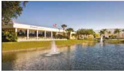
Power Systems Mfg., LLC Product Center 60Hz & E & F Class Workshop Jupiter, Florida/US
