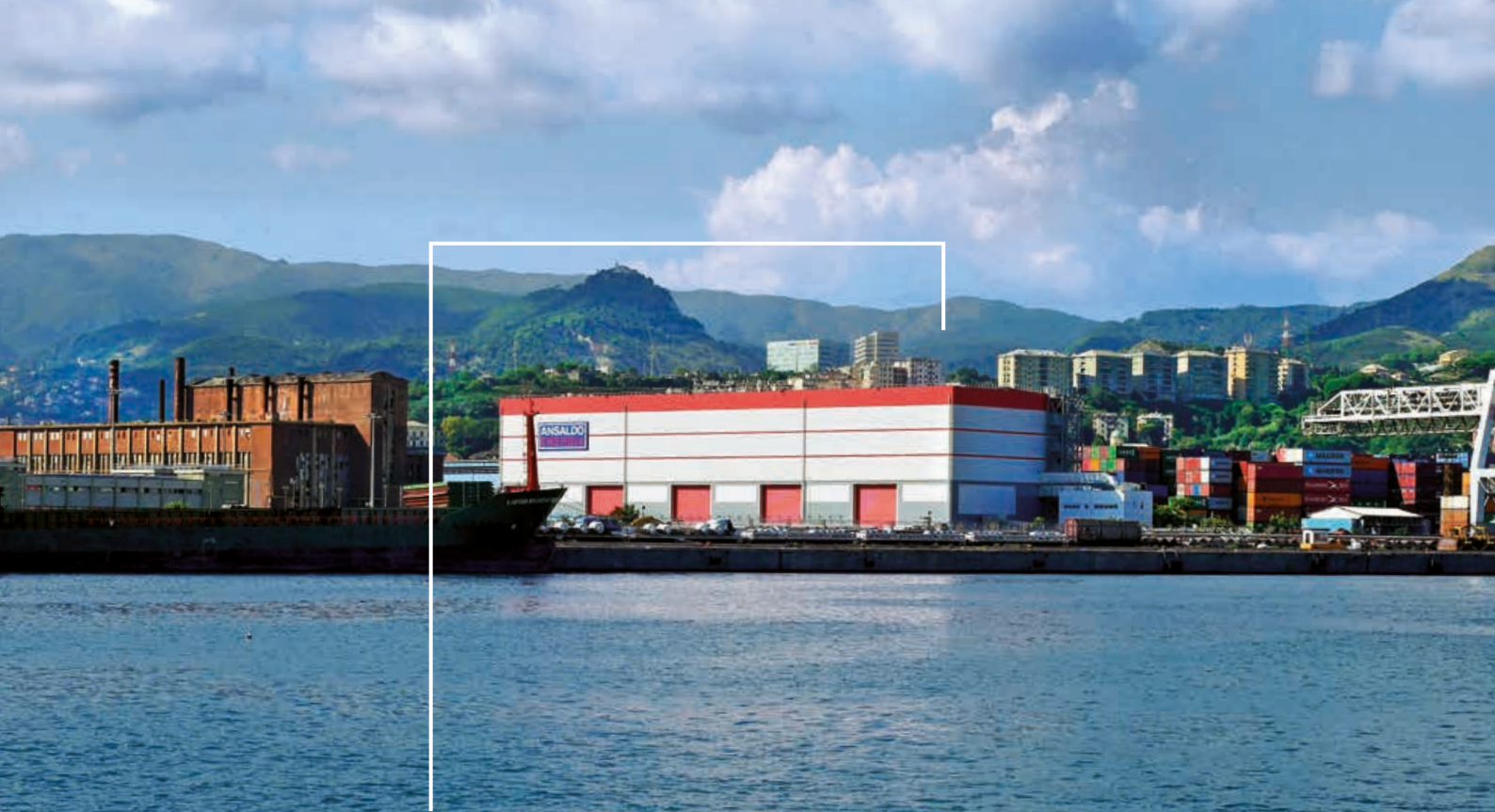
Ansaldo Energia's new plant in Genoa: large gas turbines are assembled here
